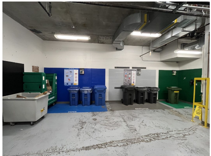
An example of a "best practice" recycling room at Marine Drive Residence. Note the bright lighting, clear separation of streams, and appropriate signage for each stream.
